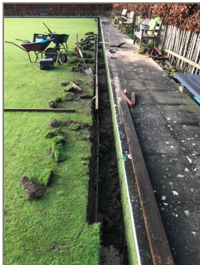
DIGGING OUT THE BOARDING AND DITCHES
